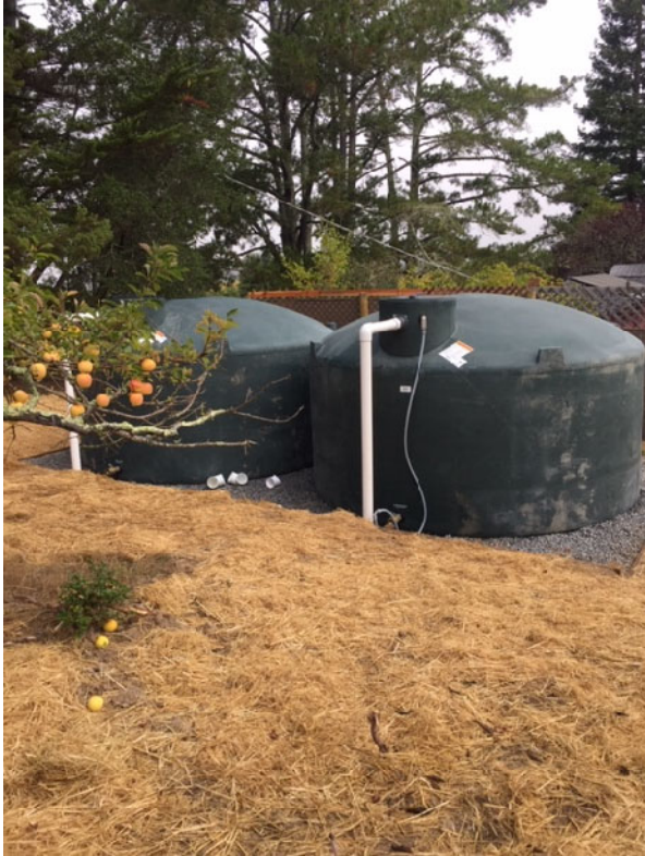
Two 10,000-gallon residential systems designed and rebated in 2022 through Phase I, which was launched in May 2022.
