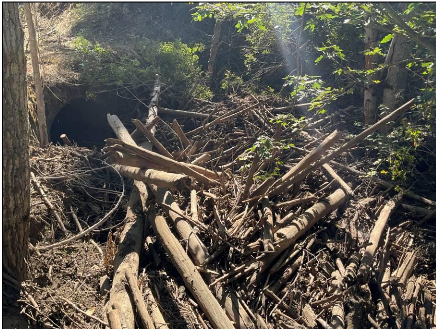
Photo 3. Woody debris deposited upstream of the culvert inlet at the Yreka Walker Road crossing on Middle Fork Humbug Creek.
