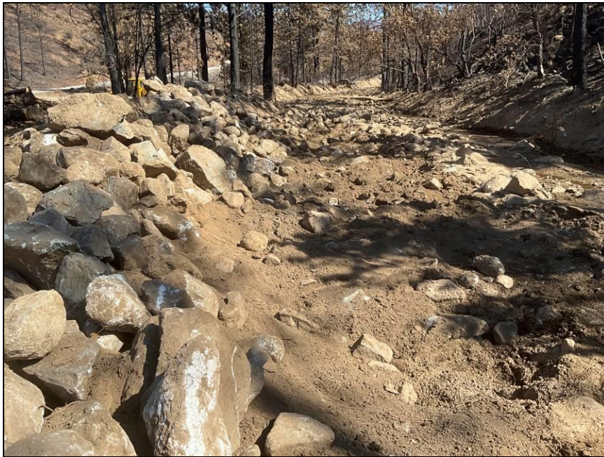
Photo 6. Photo of graded PFDF deposit in Little Humbug Creek looking upstream. A levee composed of porous PFDF deposit materials has been constructed to constrain surface streamflow and direct streamflow to the bridge crossing at Klamath River Road.
