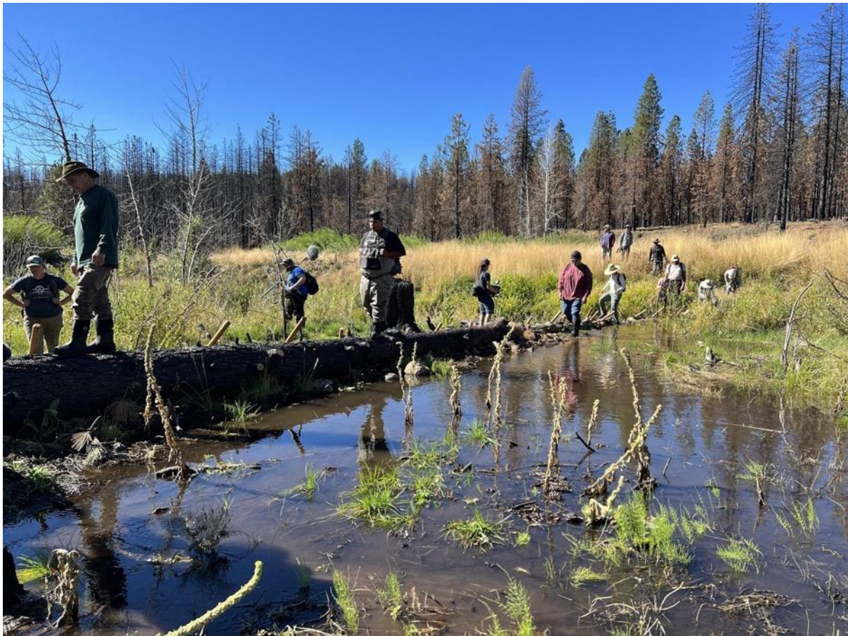
Yellow Creek – larger structures to raise water table and spread flows
