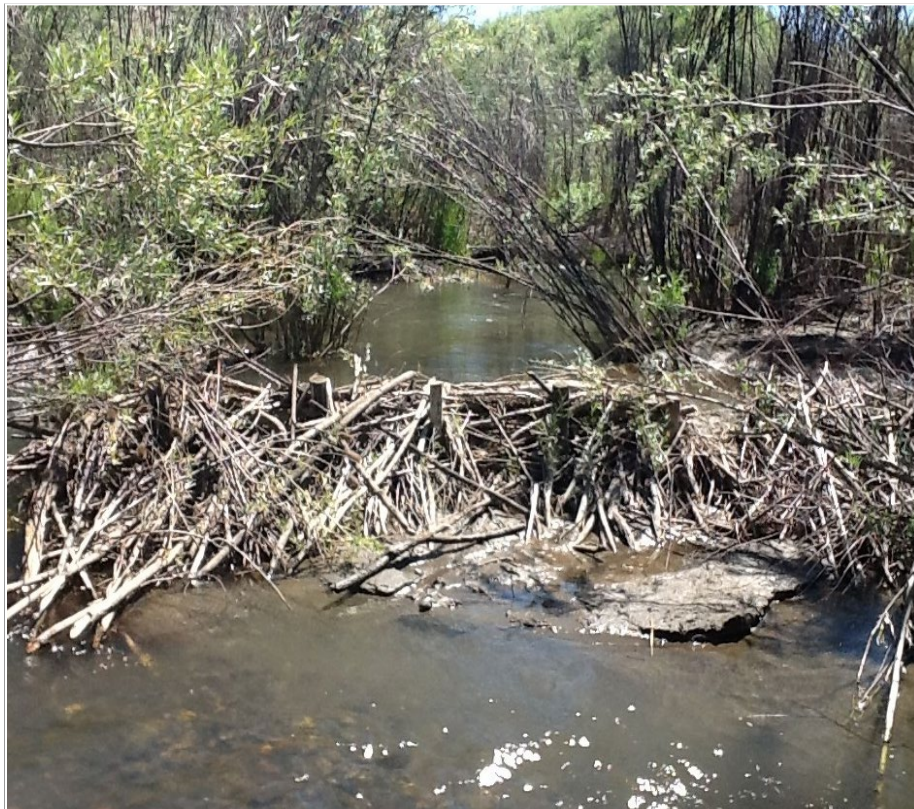
Figure 3-1: Photo of a beaver dam analog with post line and willow weave (photo from Dr. Michael Pollock)
