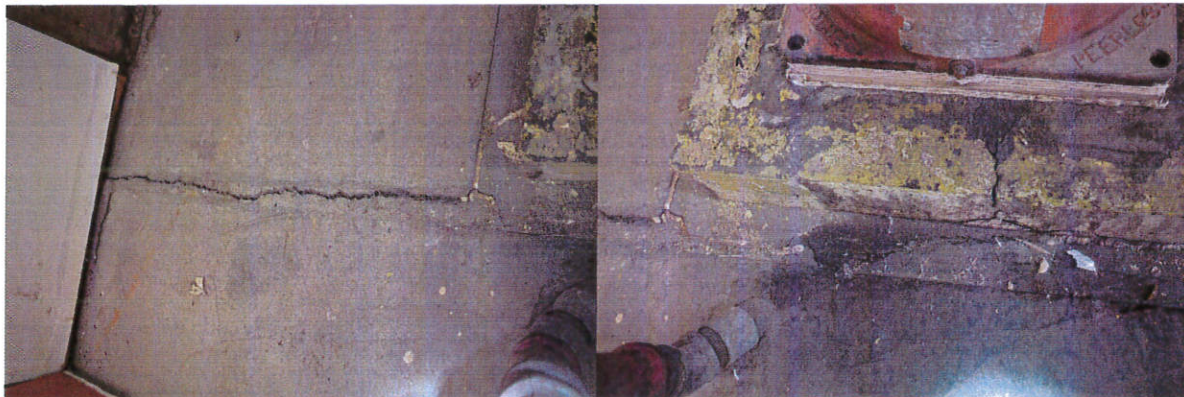
Well 6 Crack in Slab
