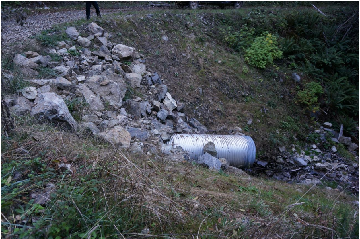
Picture 1: Recently installed culvert on B100 – example of upgraded water crossing
