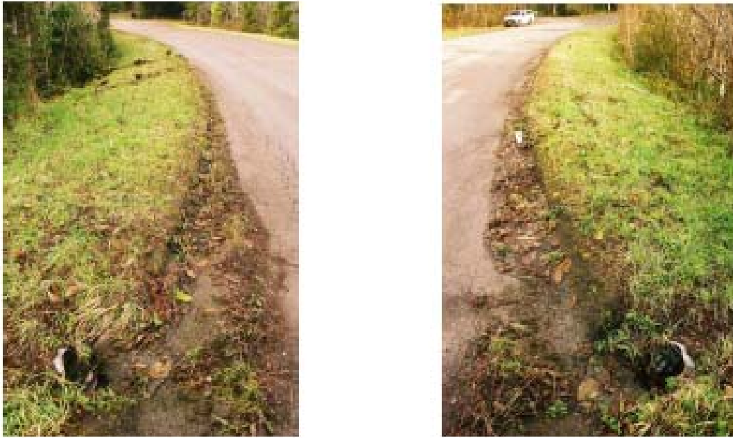
Figure 6. Photo of Westhaven Drive Looking North (photo at left) and South (photo at right) showing how stormwater is currently routed on roadway and enters culvert (bottom of photos) that drains directly to Luffenholtz Creek. Project would re-direct stormwater to utilize grassy area to provide infiltration and treatment in this area and upgradient in adjacent areas that contribute runoff.
