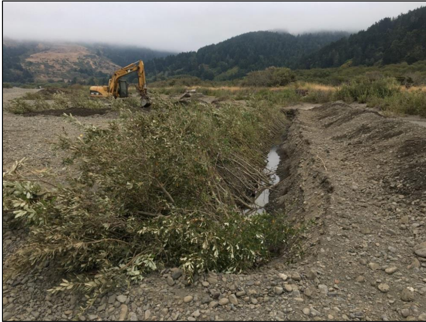
Figure 5. Example of willow baffle construction.
