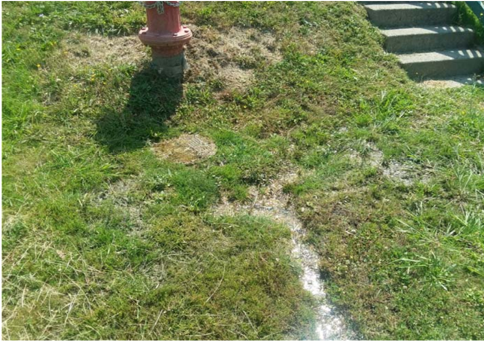
Photo 3 (Top Left) - Runoff at firehydrant located at Third Avenue and Sutter Street. Has a total chlorine residual of 0.18 mg/L and a free chlorine residual of 0.17 mg/L indicating water is from distribution system. Operators have attempted to locate the source of the leak but have been unsuccessful.
