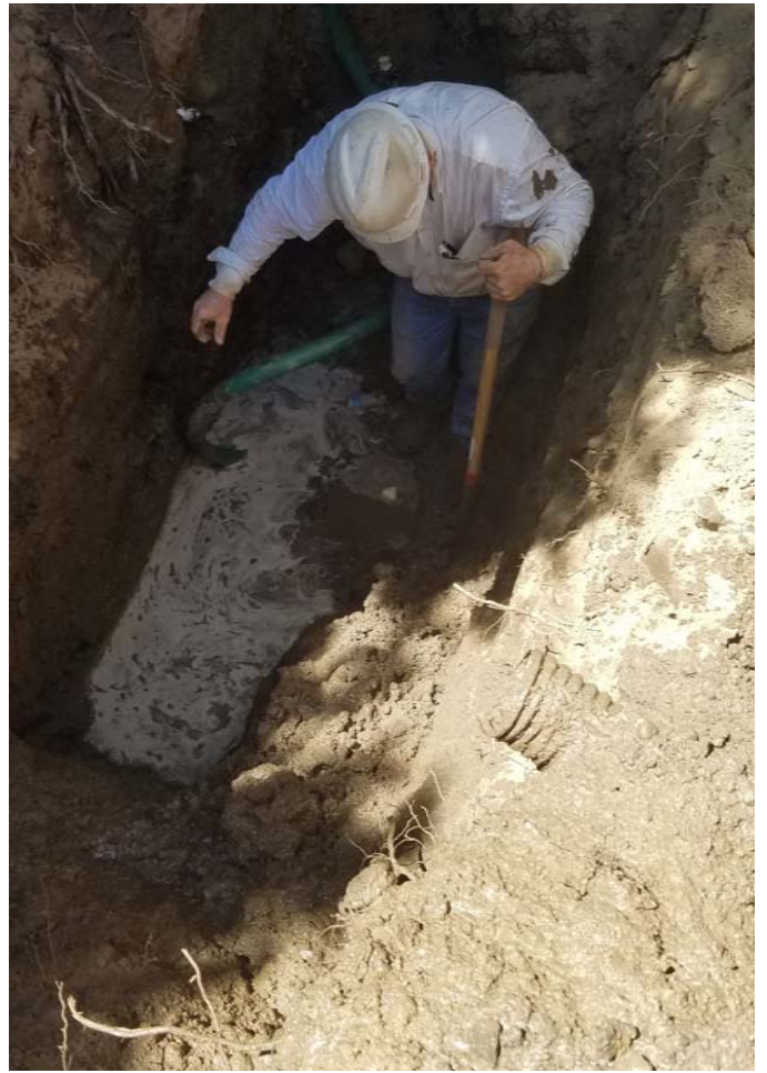
Photo 2 - Existing 4-inch AC pipe, approximately 5 feet deep, where old service line and corp stop in Photo 1 was threaded into and pulled out of AC pipe during replacement of water main.
