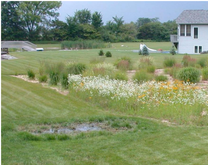
Figure 6: Effluent visible at ground surface (Lee and Wood, 2016).
