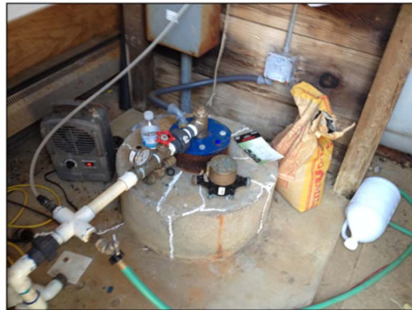
Well #2—Cap and Discharge Piping
