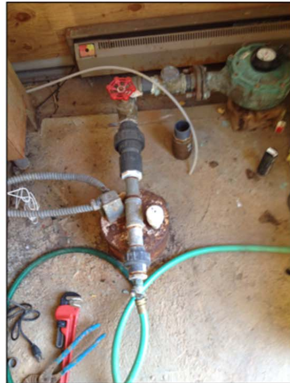
Well #1—Cap and Discharge Piping
