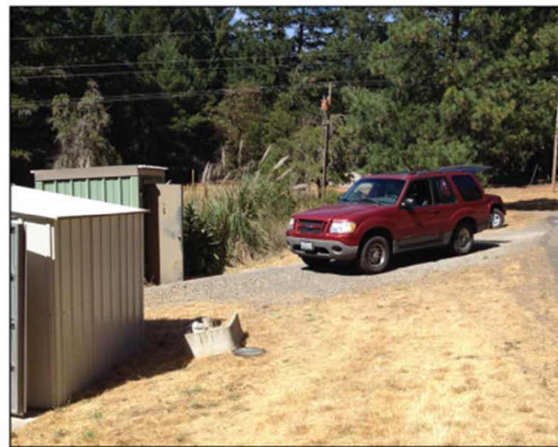
Well Houses #6 (foreground) & #1 (background)
