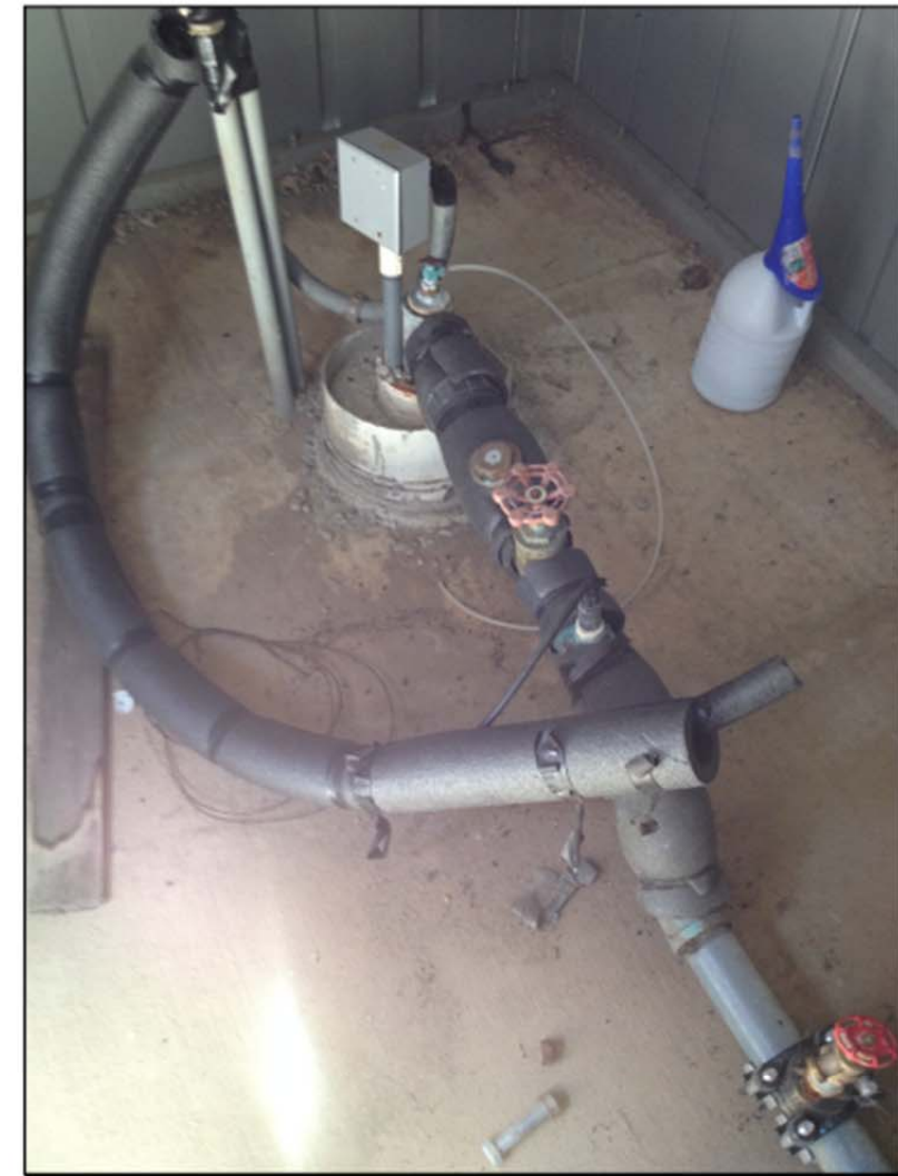
Well #6—Cap and Discharge Piping
