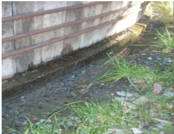
Figure 6. Leak in the redwood tank.
