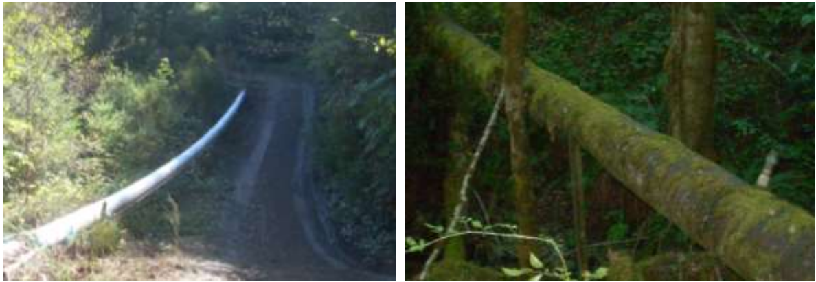
Figure 5. Severed pipe casing (left) and cable pipe bridge at slide (right).
