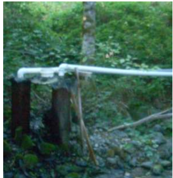
Figure 4. Supplementary intake structure.
