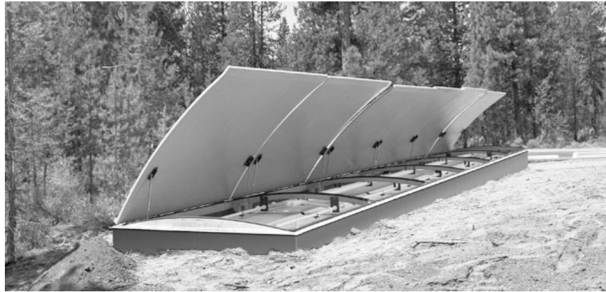
Figure 9. AdvanTex AX MAX Treatment Facility.
