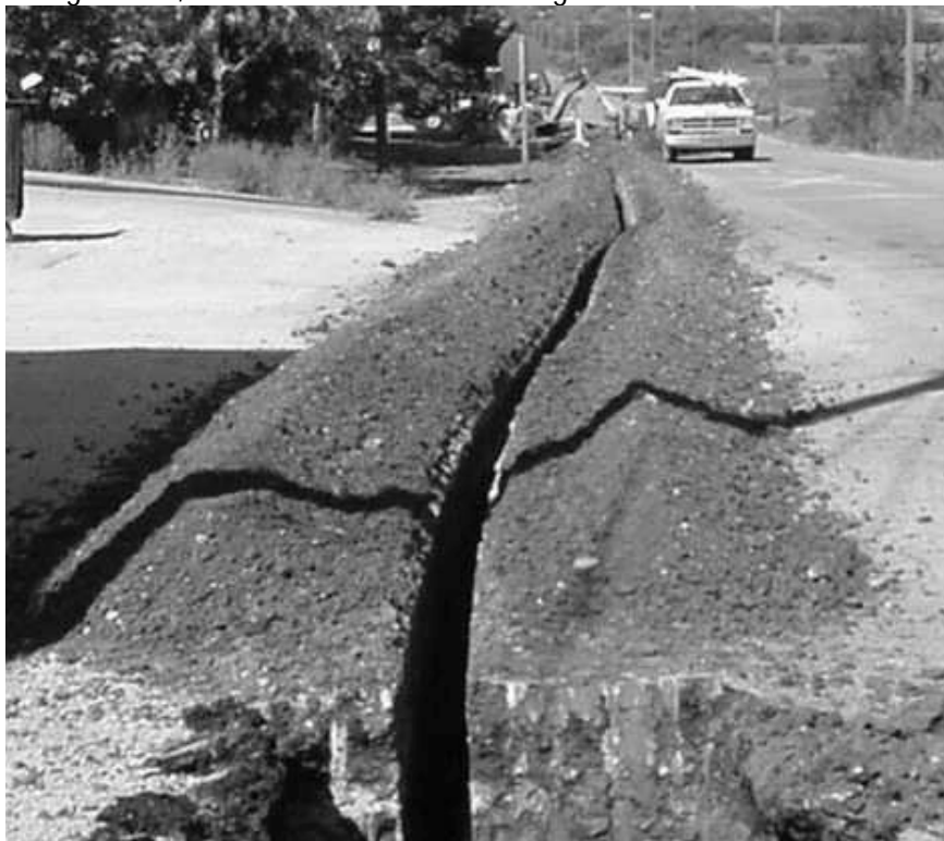
Figure 3. Typical small diameter forcemain installation.
