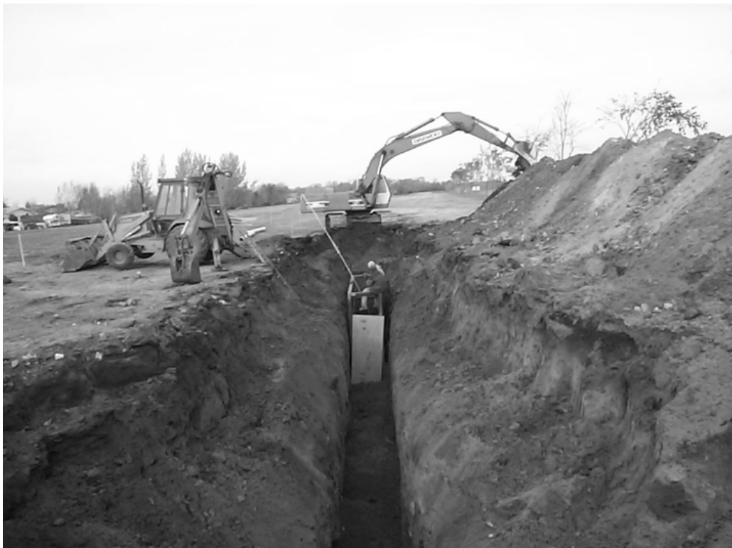
Figure 15. Typical gravity sewer main installation.
